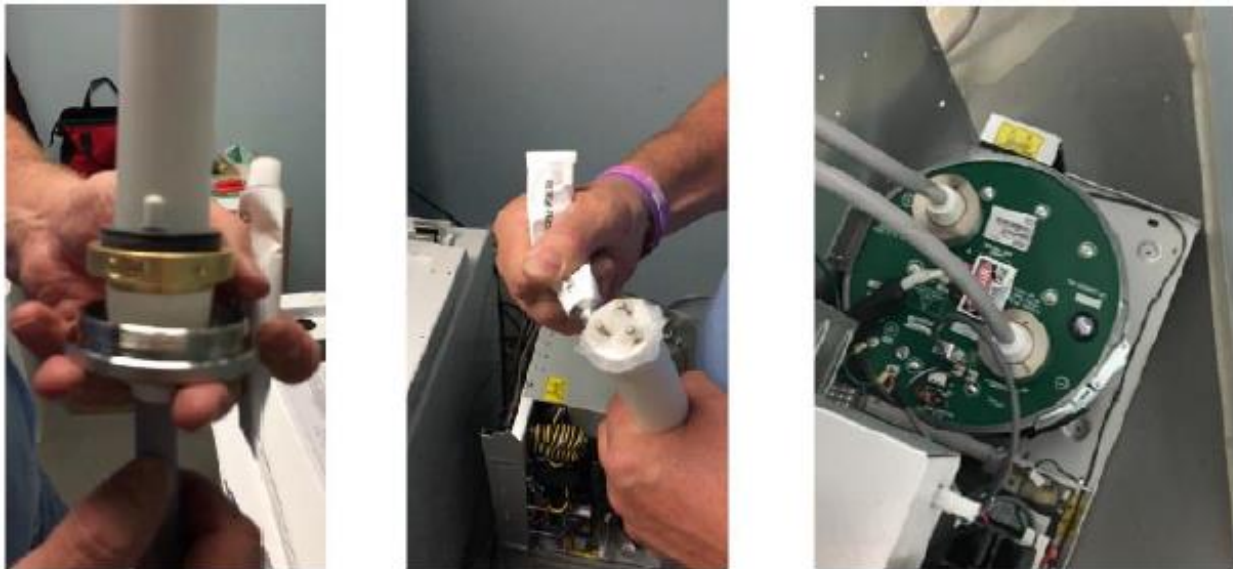
Figure 10: connecting the high tension cables to the generator
